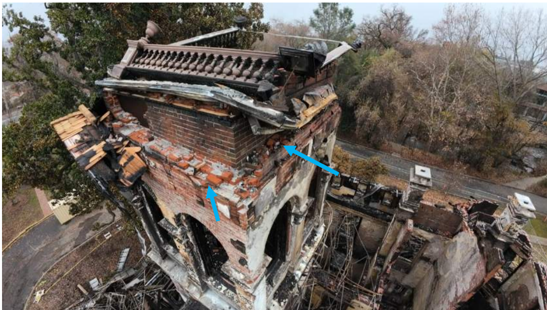
22: Exterior aerial view of the Bidwell Mansion tower. Note the extensive damage that occurred to the brick, not only where the section of low wall collapsed, but also where attached wood materials damaged brick while collapsing (blue arrows).
