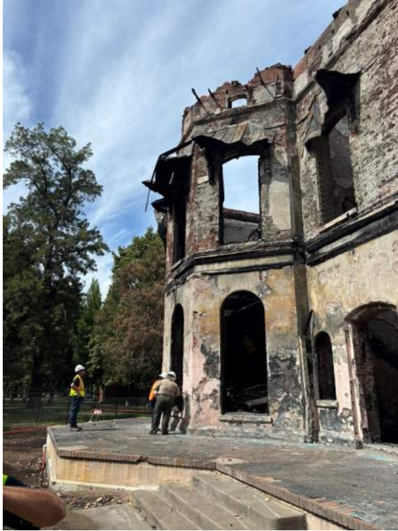
07: View from north looking east, 09.09.25.
