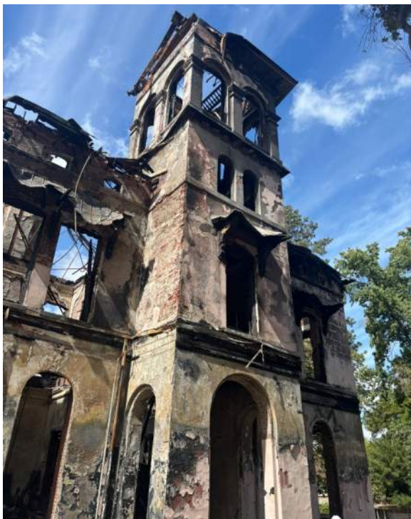
02: Primary (east) elevation view of tower from south, 09.09.25.
