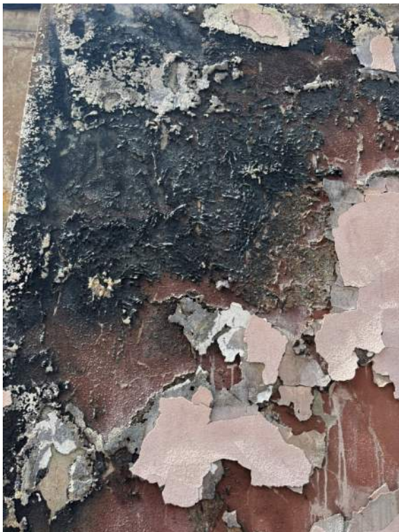
06: Typical cement plaster finish, 09.09.25.
