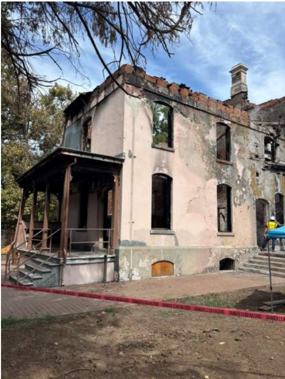
16: Kitchen and rear (west) porch, 09.09.25.
