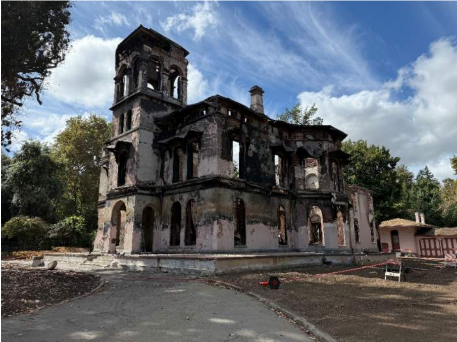
18: Bidwell Mansion remains looking Southwest.
