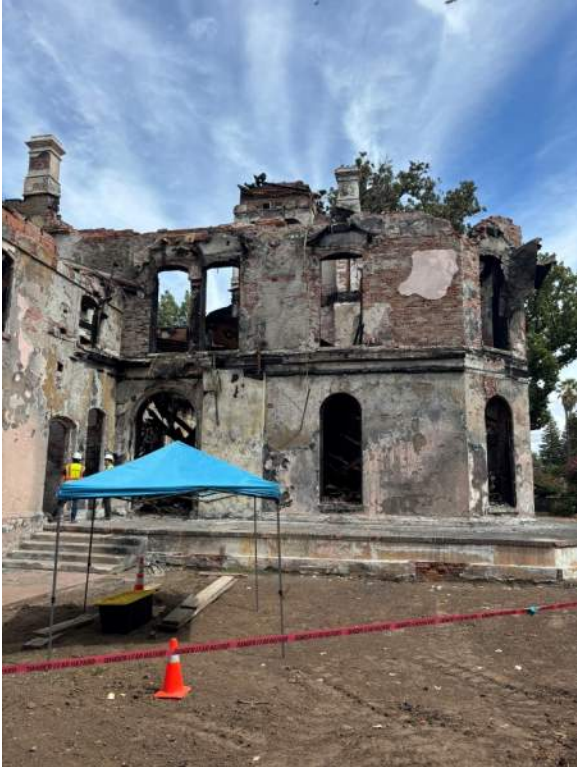
15: West elevation conditions, 09.09.25.
