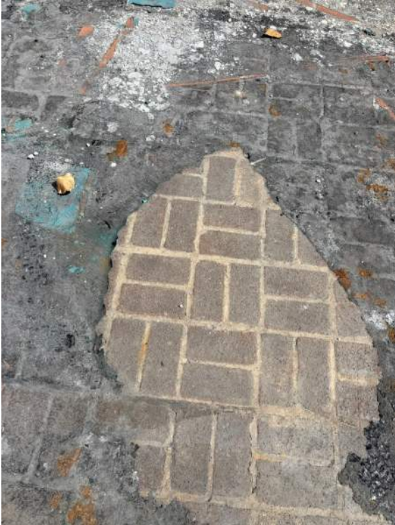
11: Flooring protection adhered to brick porch face, 09.09.25.
