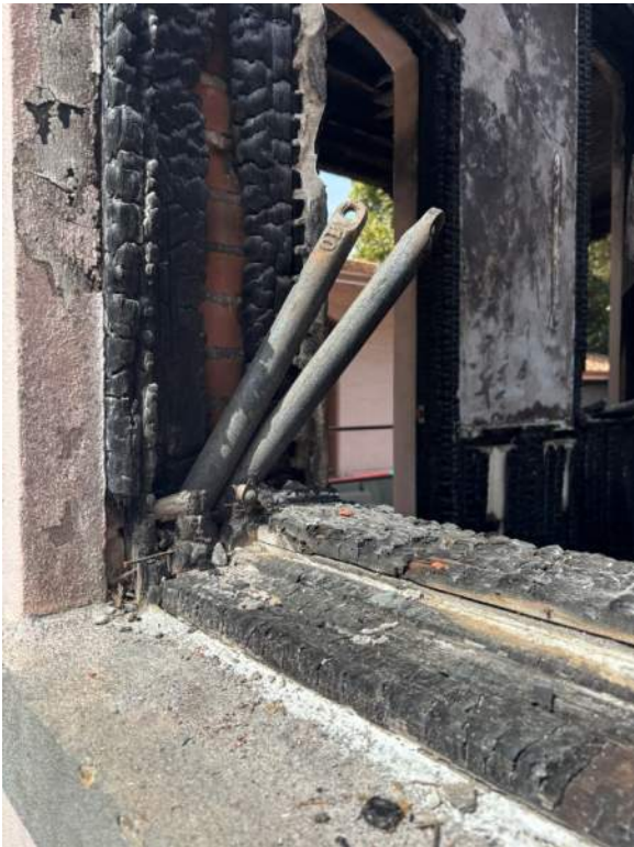
10: Typical window frame and sash weights, 09.09.25.
