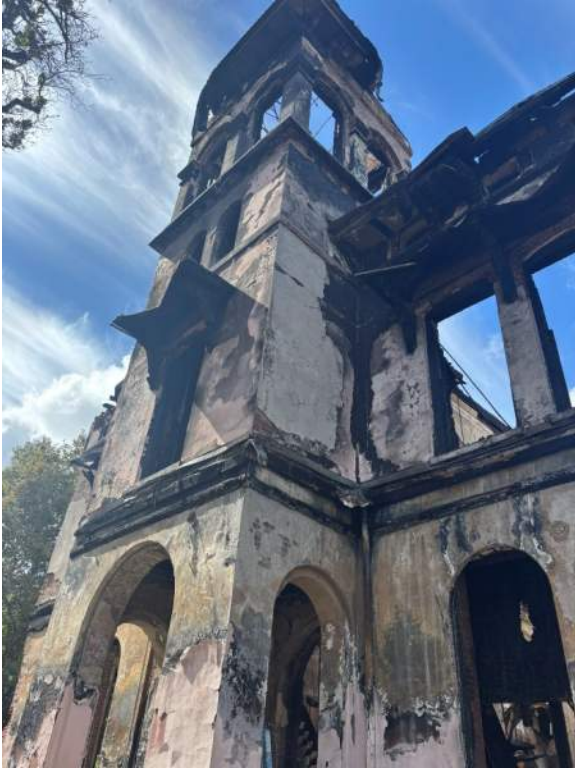
03: Primary (east) elevation view of tower from north, 09.09.25.
