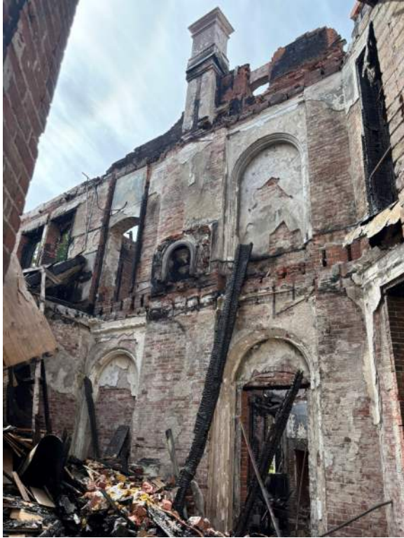
13: Building interior conditions- intact fireplace surround, 09.09.25.
